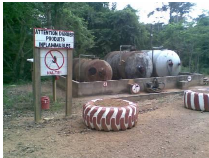
Figure 33 — Fuel tanks must be placed within a concrete bund to prevent spills and reduce fire hazard (Photograph P. van der Hout)
