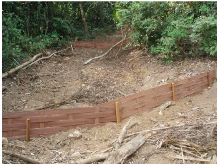
Figure 44 — Siltation barriers on skid trail made from sawmill waste (Photograph P. van der Hout)
