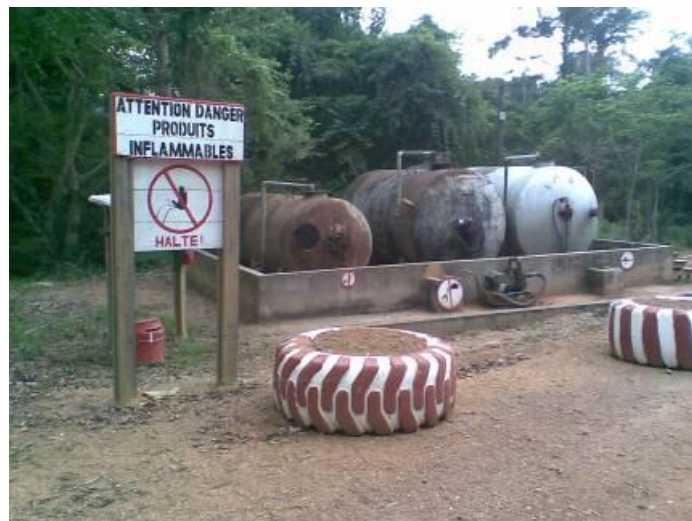
Figure 49 — Fuel tanks must be placed within a concrete bund to prevent spills and reduce fire hazard (Photograph P. van der Hout)
