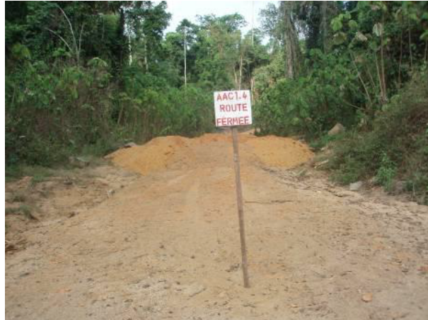
Figure 46 — Road barred by means of a trench dug across the road (Photograph P. van der Hout)
