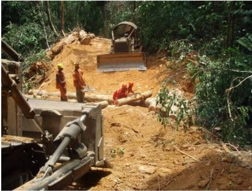
Figure 31 — Construction of a “Japanese” culvert (Photograph P. van der Hout)
