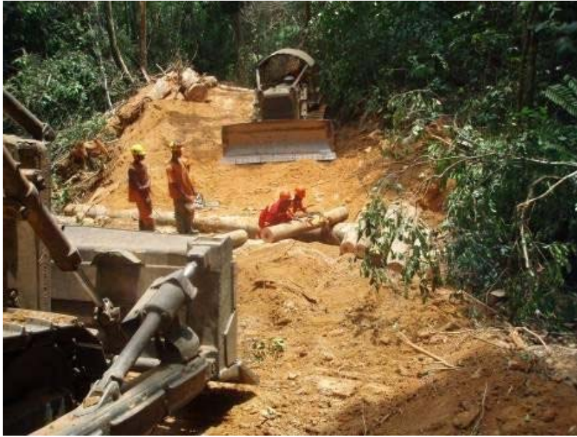
Figure 17 — Construction of a “Japanese” culvert (Photograph P. van der Hout)
