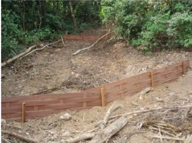
Figure 29 — Siltation barriers on skid trail made from sawmill waste (Photograph P. van der Hout)
